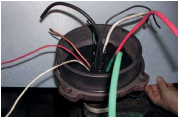
7. Pour the potting compound to the final level and make sure the leads are separated.
